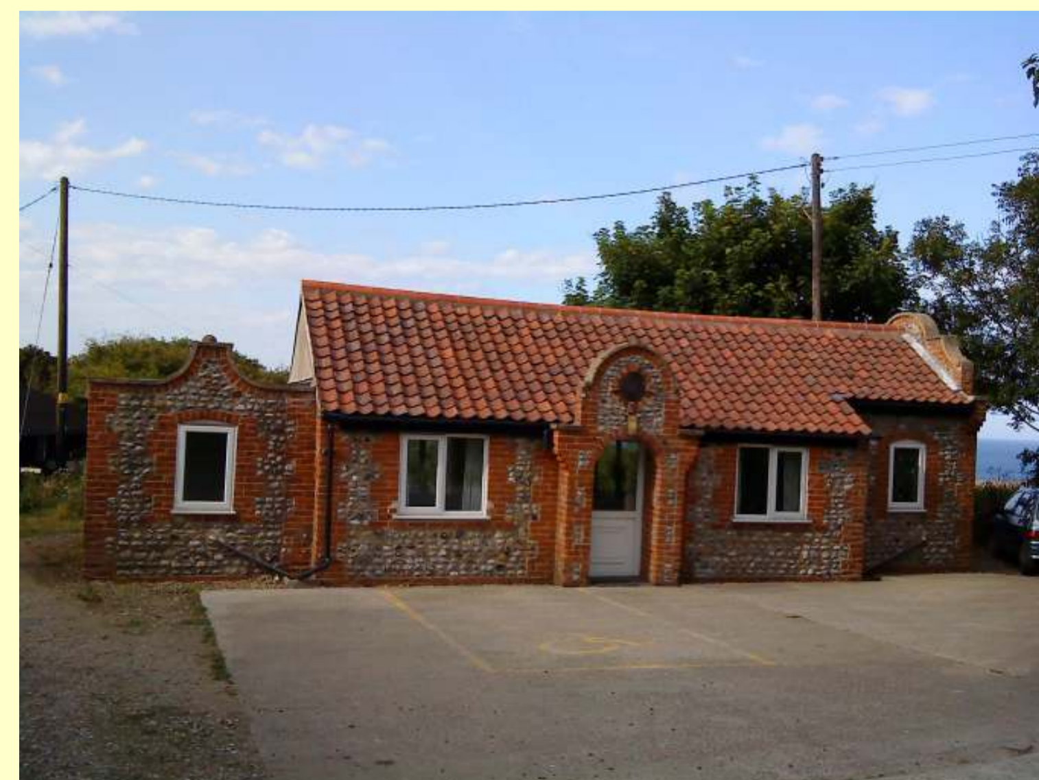
Pilgrim Shelter - built using local materials
