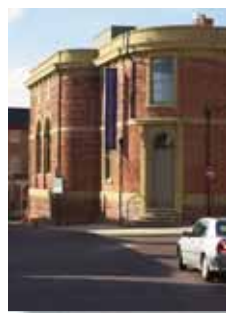
Cinema has returned to Fakenham in the newly refurbished Corn Exchange
